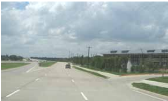
Existing development along S.H. 114
